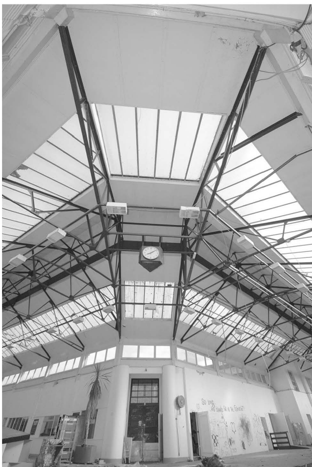
Fig 5. The interior of Northampton Fishmarket showing the steel roof trusses and the three-sided clock.
