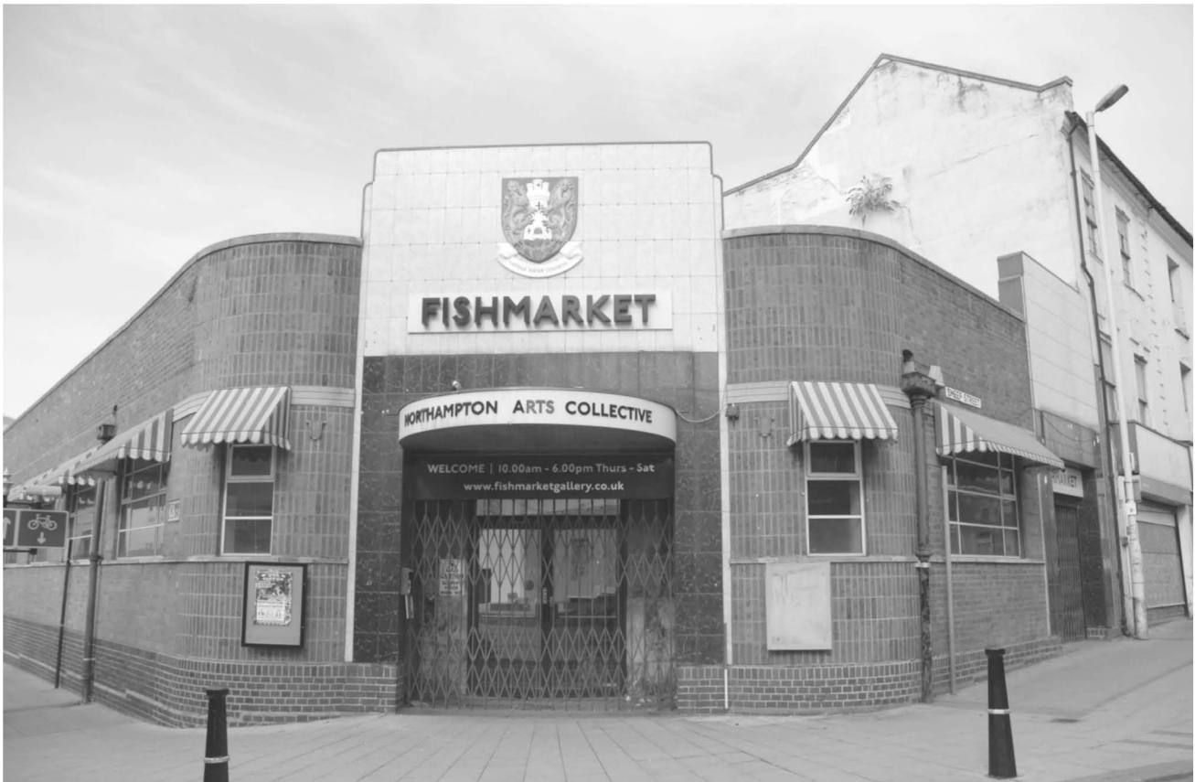
Fig 4. The main entrance to Northampton Fishmarket showing the Art Deco tiled surround.
